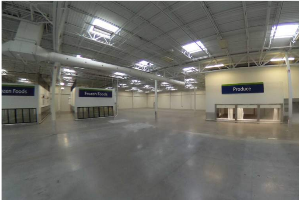
Auto Lab area prior to renovation - 2019
